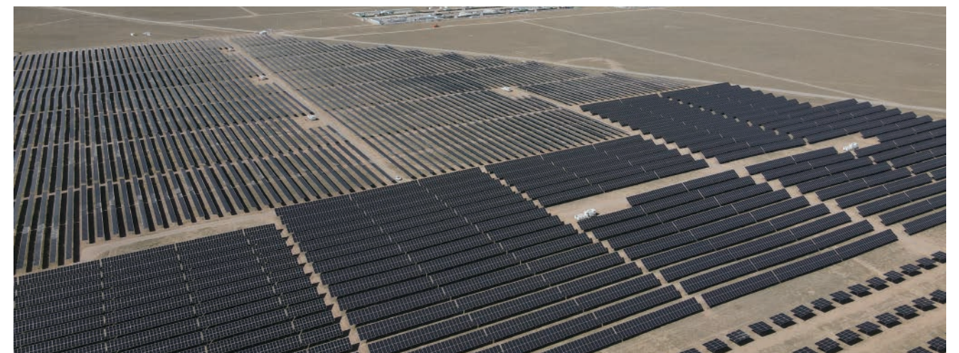
Qinghai, China Completed: 2024
